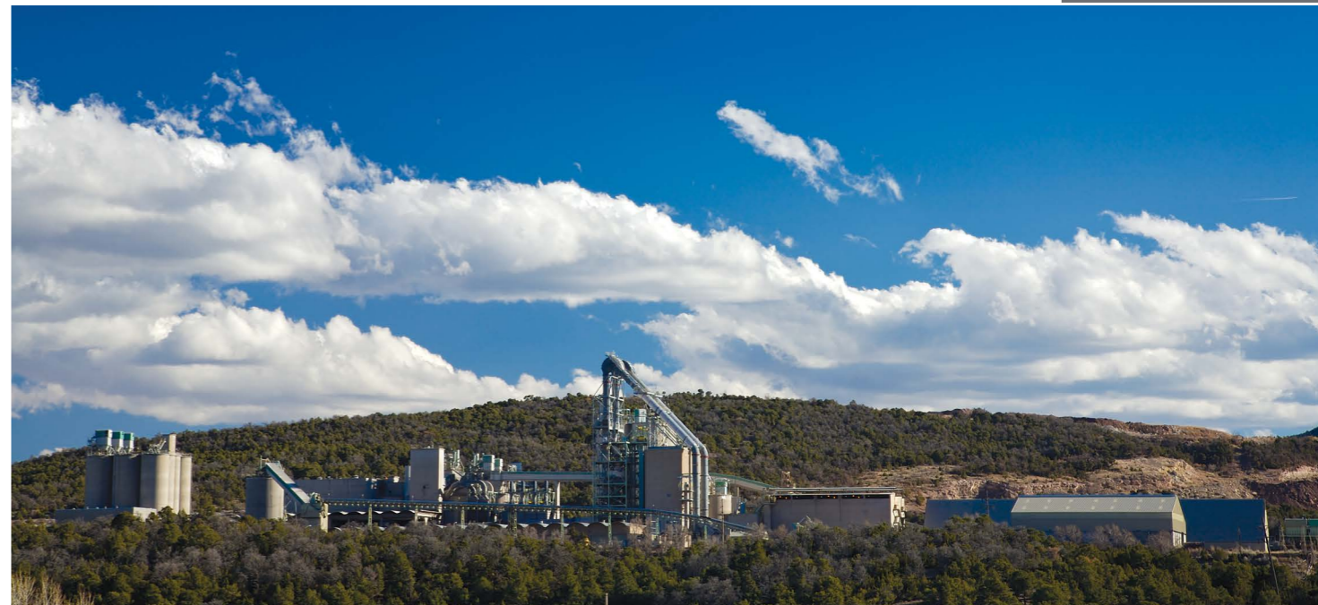
The Tijeras Plant in Albuquerque, New Mexico.
